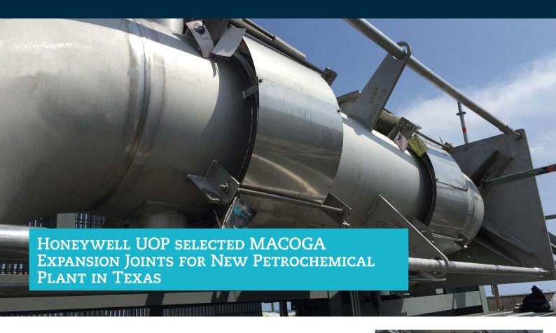
We have completed the detailed engineering, manufacturing, testing and shipping of a large number of high-tech expansion joints (Universal Tied, Double Hinged, Double Gimbal and
